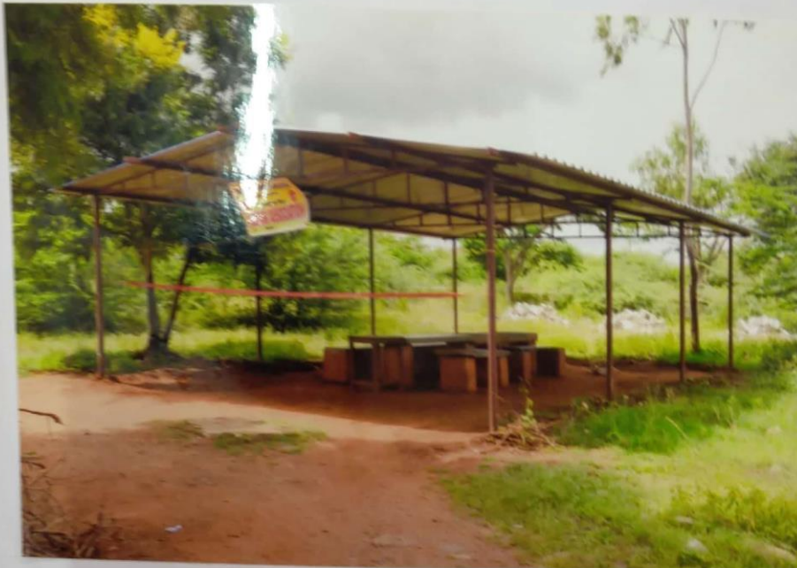
Construction of canteen ready for inauguration.
